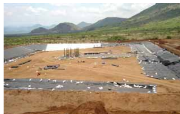
ASA Metals Pty., Ltd. build bedding on the gangue dam to prevent penetration and protect the underground water.
