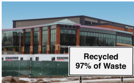
To date, the construction of the Feynman Center has recycled 97% of its waste.
