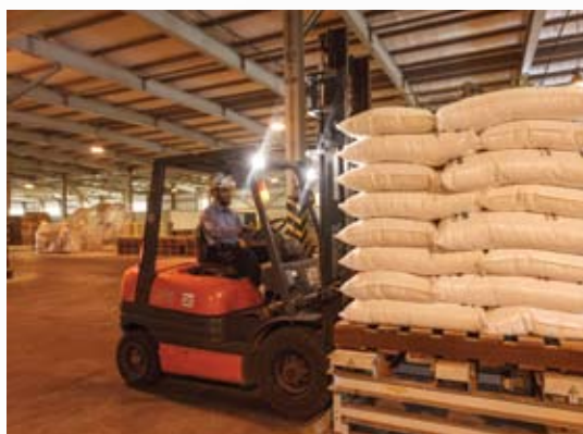
Urea Bagging Unit
