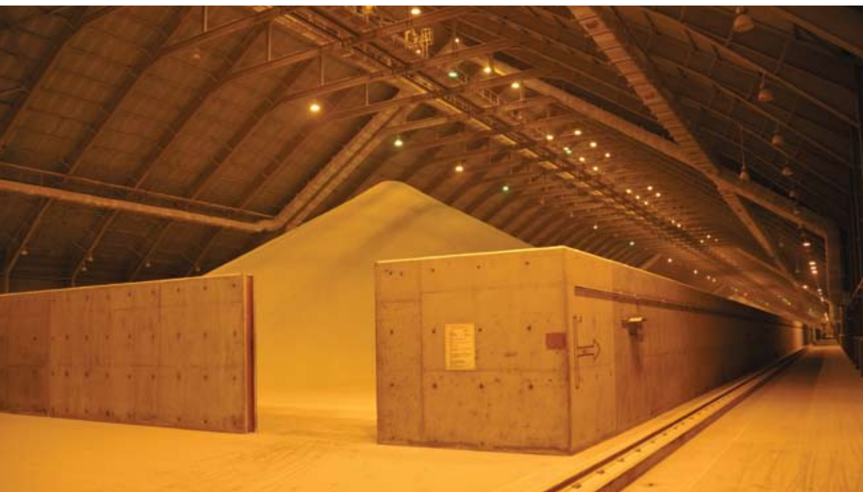
Urea bulk storage warehouse
