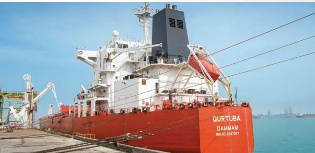
Ammonia / Methanol ship loading facilities
