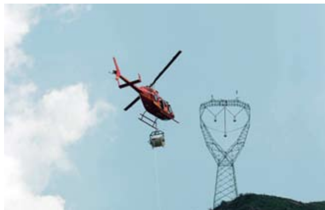
Placing leading string in the air, and alleviating damage to the nature
