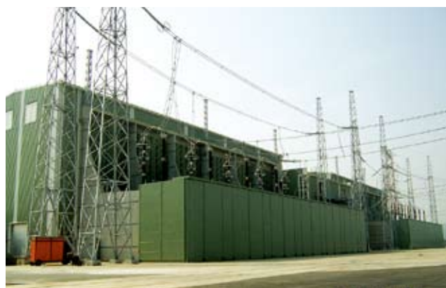
Barriers are used in converter stations to absorb noises
