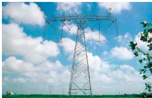
500kV double-circuit line on the same tower
