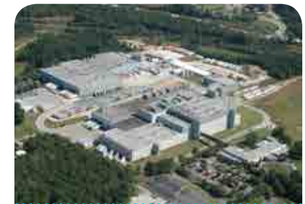
△ Our Big G plant in Covington, Georgia, first piloted the energy reduction process, decreasing the energy use rate (per pound of production) by 29 percent and saving an estimated US$5 million in energy over five years.
