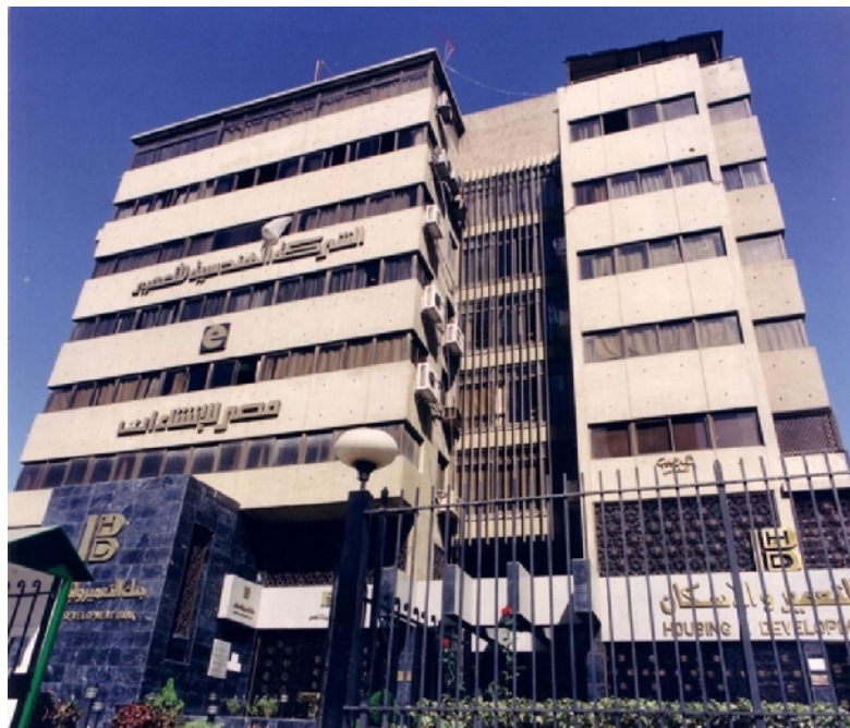
Encon Administration Building
