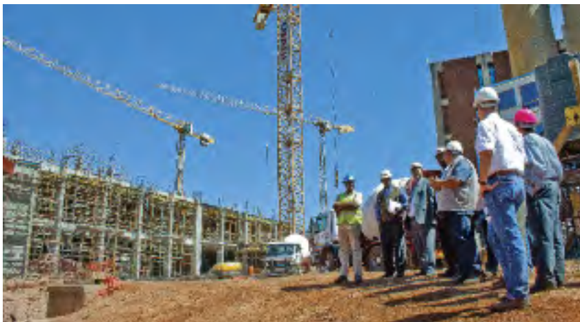
Building at the Florida Campus continues apace.
