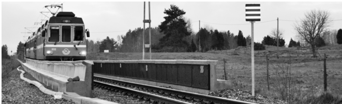
Trackside noise-reduction barriers reduce noise – effectively, cheaply and without affecting the landscape.
