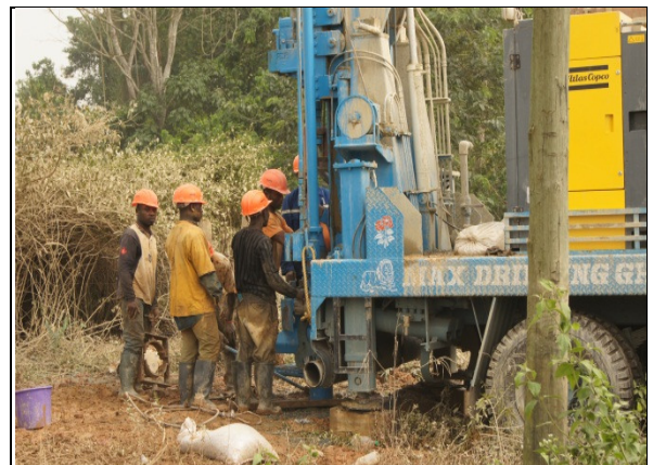
Plate 54: Borehole under construction at Akyem
