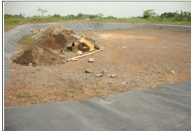
Plate 9 shows volatilization pad under operation.
