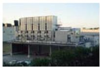
Effluent gas treatment equipment (Fukuoka Plant)
