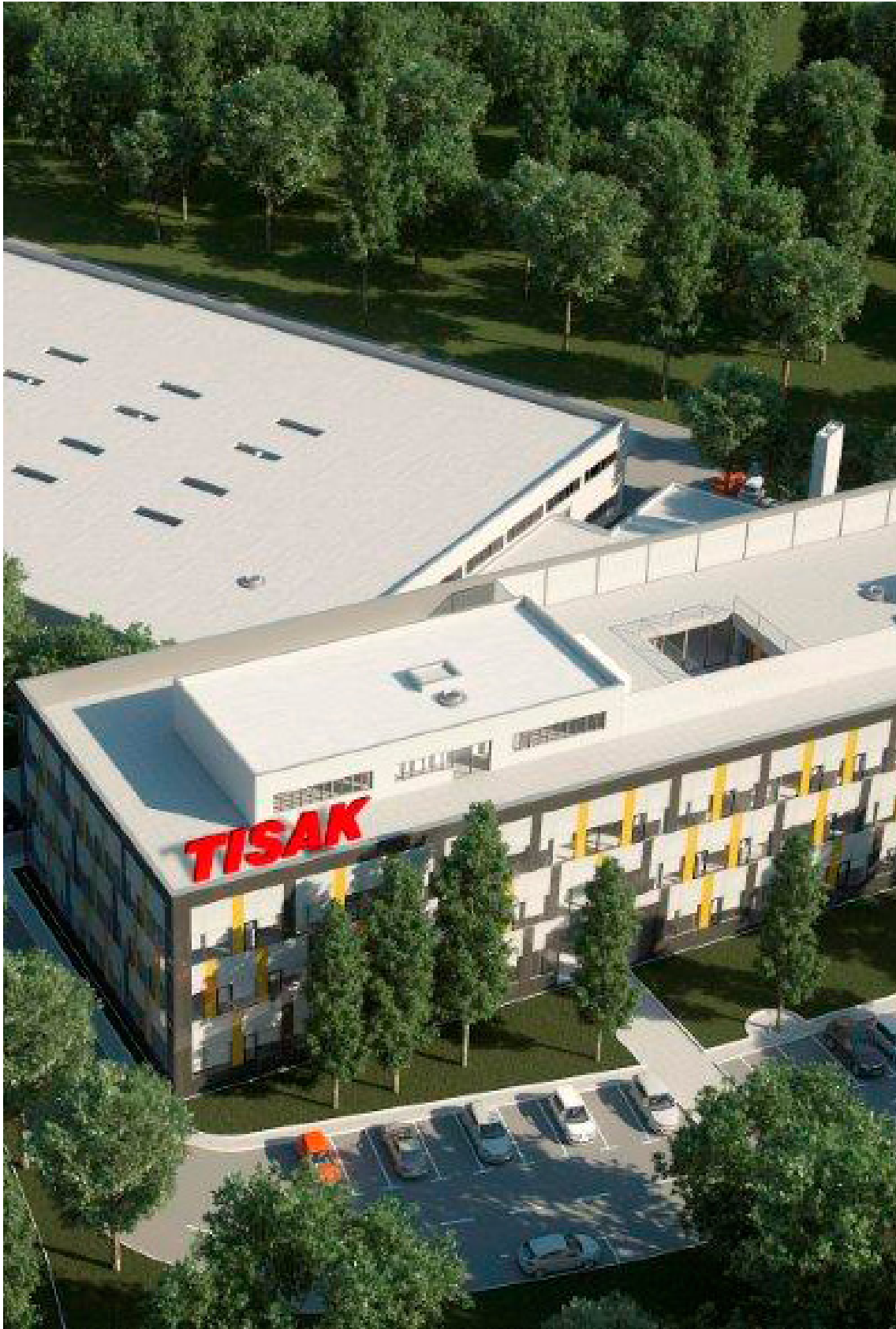
Tisak Distribution Centre
