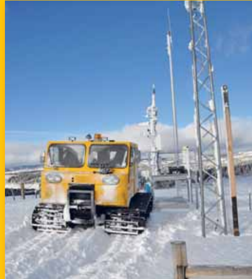
Maintenance work on some customer sites require special equipment for working in deep snow.
