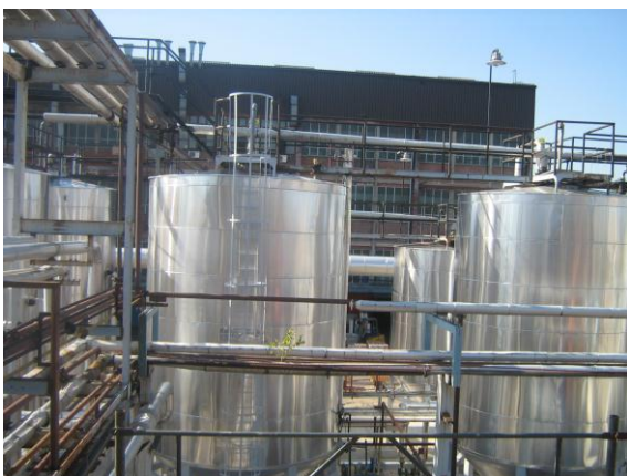
New insulation on inside storage tanks
