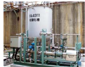
Sludge micro-solubilization treatment (Osaka Works)
