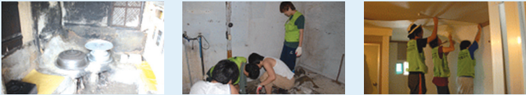
Broke down the old kitchen, and replaced the wallpaper, linoleum, and sink, and renovated it into a stand-up type kitchen
