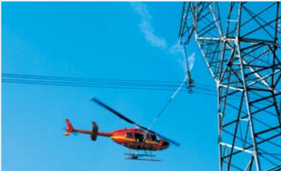
Insulator Cleaned with the Application of Helicopter
