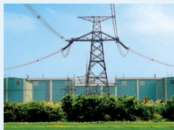
Soundproof-wall of Converter Substation
