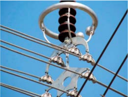
Fittings for UHV Transmission Lines
