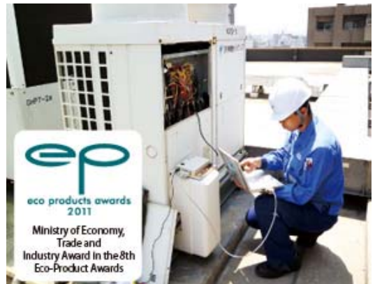
VRV Energy-Saving Tuning is one way to save energy. By having the control panels of their existing air conditioners' outdoor units tuned, users can save up to 20% in energy.
