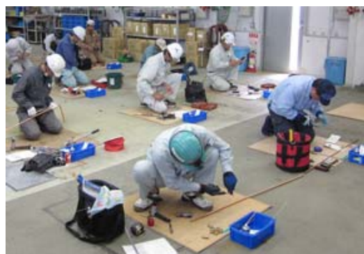
Refrigerant pipe installation training
