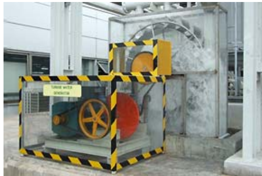
Hydropower utilizing cooling water from the plant
