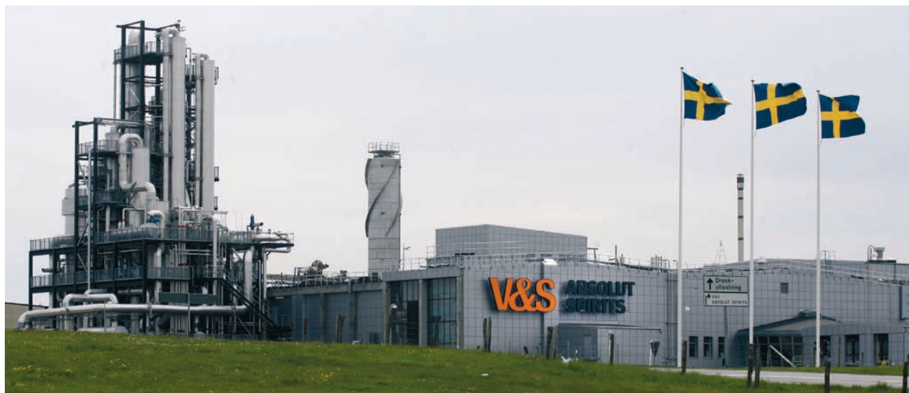
The distillation plant in Nöbbelöv, Åhus, Sweden, is one of the world's most energy-efficient plants for the production of crude alcohol and rectified alcohol.
