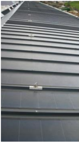
Anchor points for prevention of falls attached to Trimo EcoSolar panels
