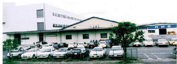
Clean-up work has been completed at the Ichinoseki Plant
