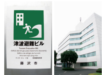
One of the Fujisawa Plant buildings available as a tsunami shelter
