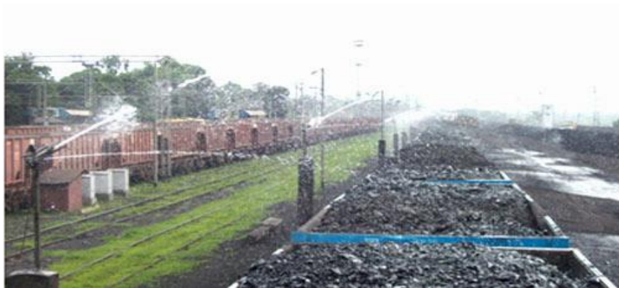
Static Sprinkler at RCM siding of Piparwar Area of CCL
