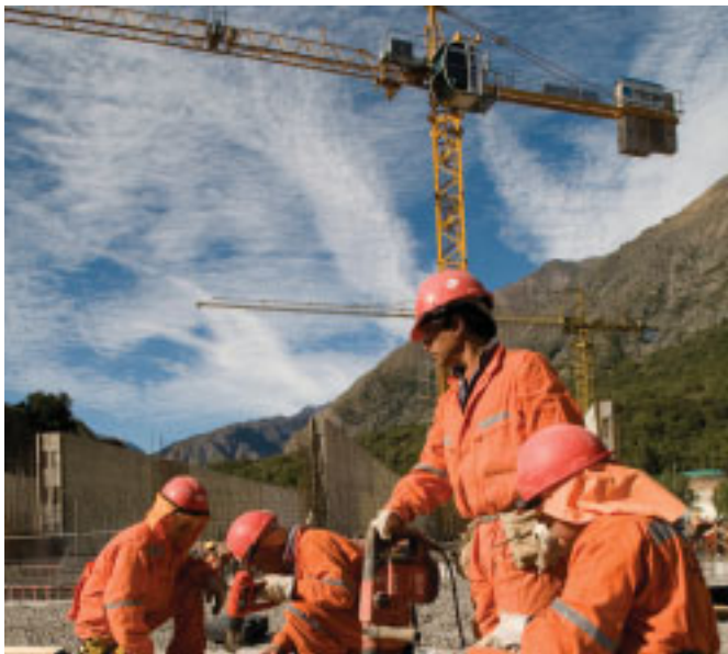
CONSTRUCTION WORKERS IN CHILE
