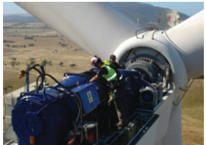
GEARBOX CHANGEOUT AT CHALLICUM HILLS WIND FARM, AUSTRALIA
