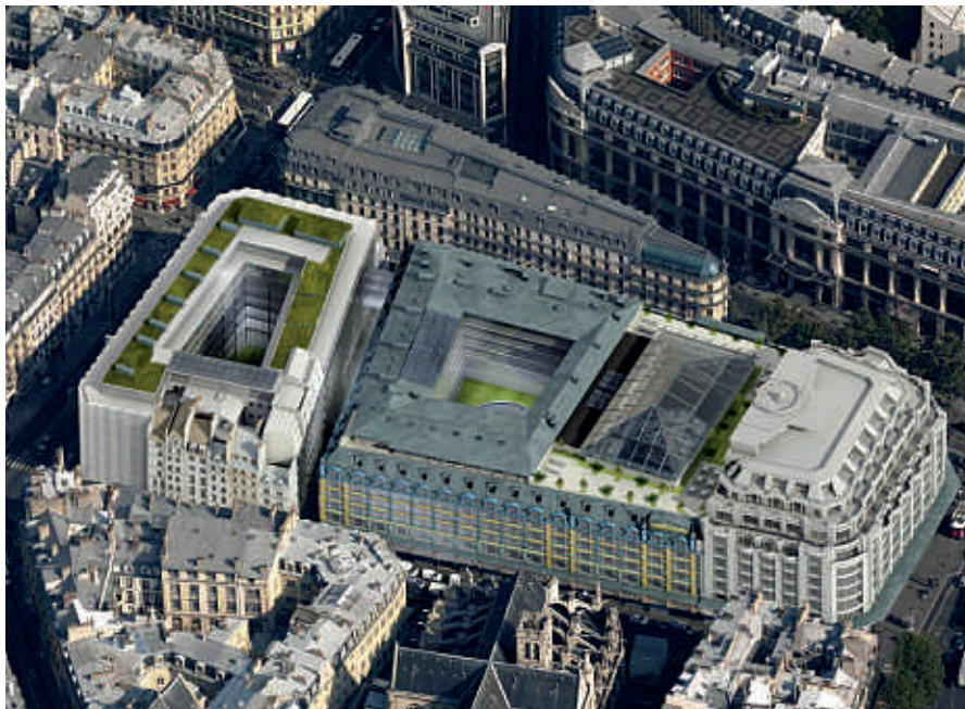
Aerial view of the future Samaritaine.
