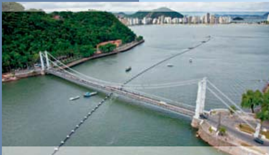
Dragging the Sea Outfall - Praia Grande
