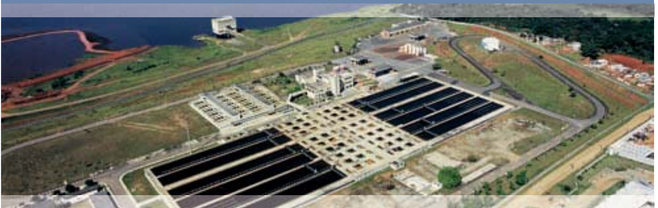
Water Treatment Plant - Taiapuêba
