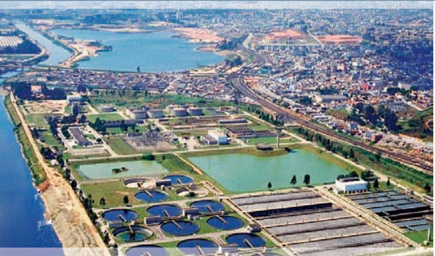
Barueri Sewage Treatment Plant
