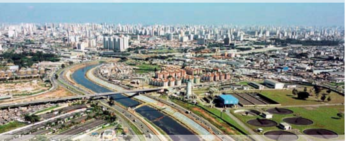
Parque Novo Mundo Sewage Treatment Plant next to the Tietê River
