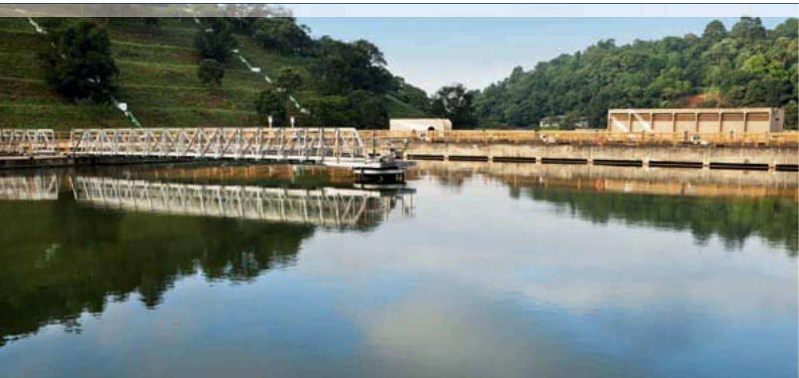
Guaraú Water Treatment Plant
