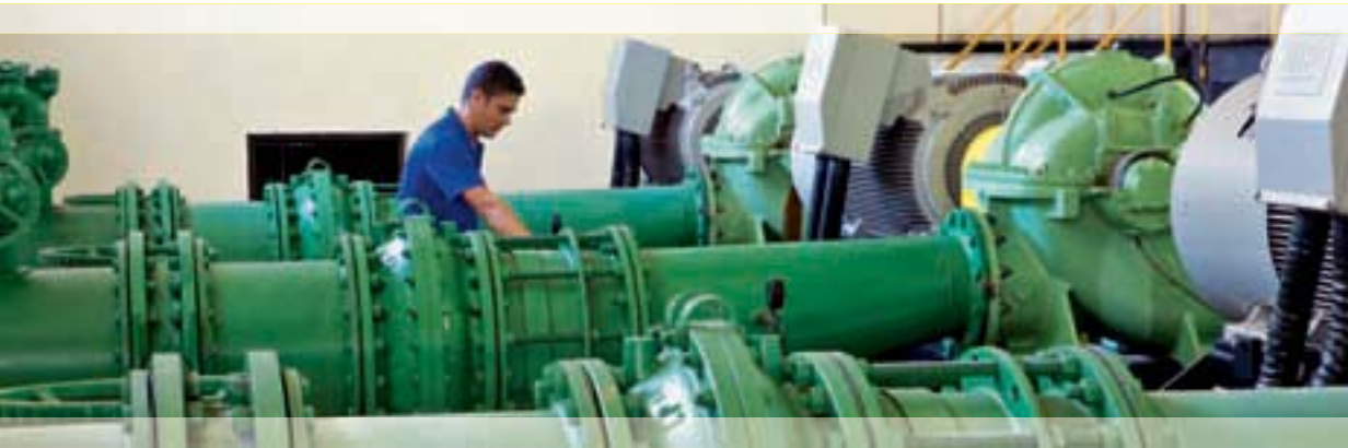
Water Treatment Plant - Alto Cotia
