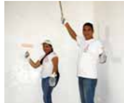
Employees help to restore the school
