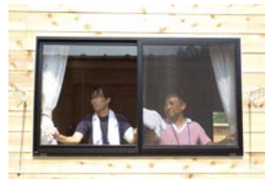
Fitting heat shielding films
