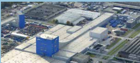
nkt cables' plant in Cologne, Germany
