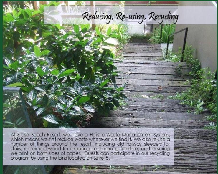
Outdoor stairs from railways wood
