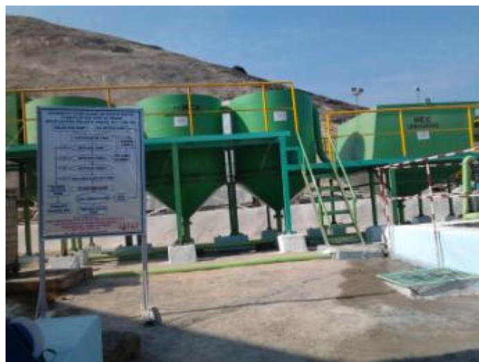
Wastewater treatment plant for tunnel wastewater
