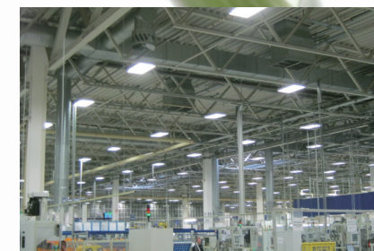
Installation of high energy efficiency lights at Czech Plant
