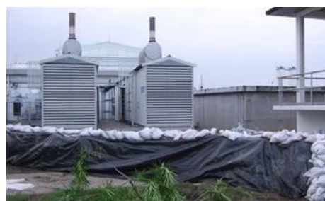
A levee built to prevent flood water from reaching the facility
