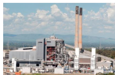
Oxyfuel combustion boiler at the Australia Callide-A coal-fired power station in Queensland, Australia
