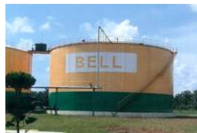
The anaerobic biogas digester, recovering methane from the effluent
