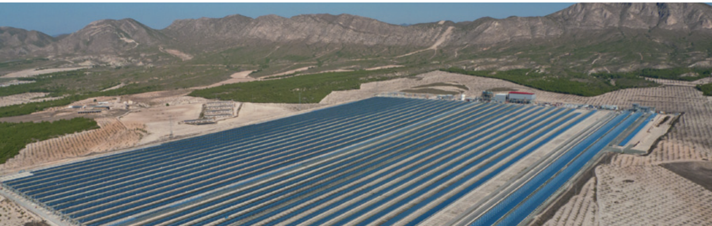
The Puerto Errado 2 solar thermal power plant (Murcia) is the largest plant built to date using direct steam generation technology based on Fresnel-type linear collectors on a commercial scale (30 MW). OHL Industrial has introduced significant innovations in the technology to make its operation feasible.
