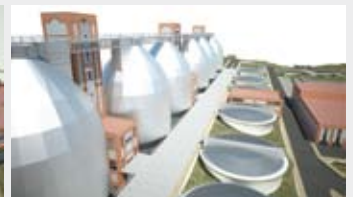
| Sludge digestion tanks
