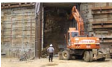
| Construction site using the pressurizing support tunnel method
