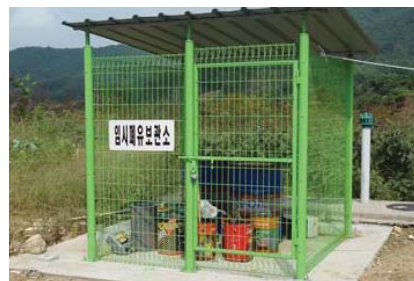
Temporary storage for waste oil
