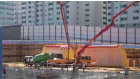
Noise-control facilities: Noise-proof walls and balloon-shaped noise-proof walls
