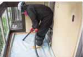
Finish asbestos removal
