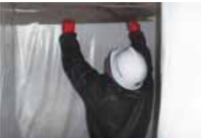
Prepare for asbestos removal
