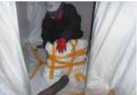
Remove and seal asbestos
