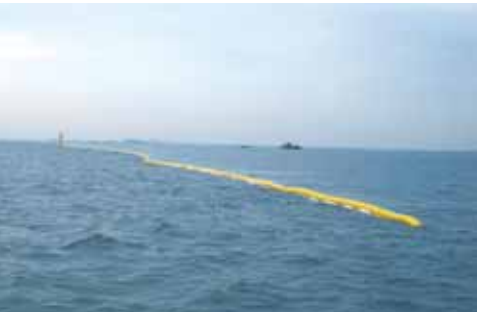
Installing Pollution-Containing Fences around Construction Sites
