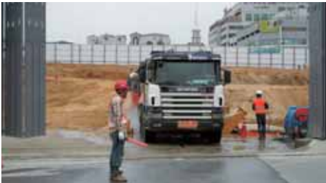
Dust-control facilities: Wheel washers
