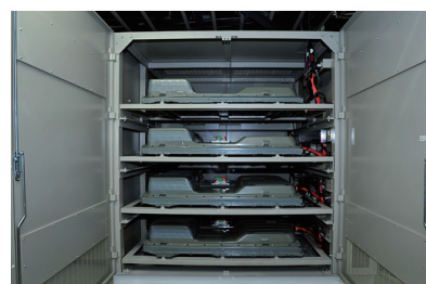
The energy storage system holds the equivalent of four Nissan LEAF batteries.
