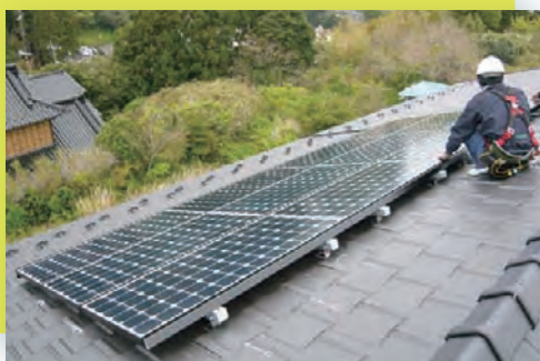
Installation of a photovoltaic power generation system (evacuation center in Kesennuma City)
