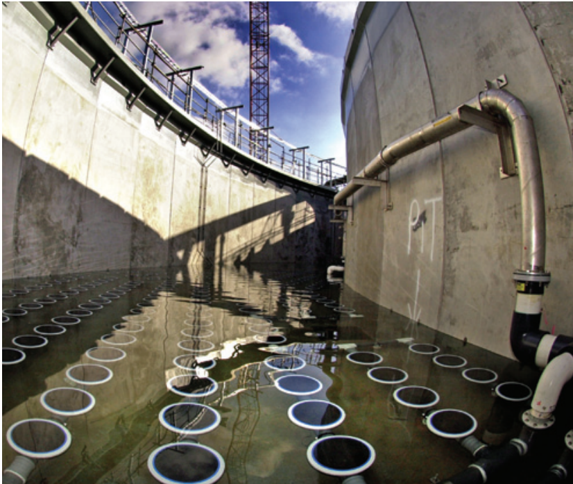
Gippsland Water Factory
