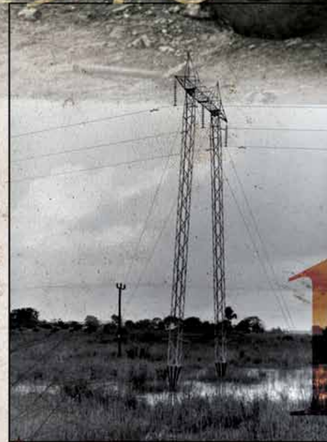
132kV line structure and 33kV line across Ruiru at the start of long rains - 1963.
