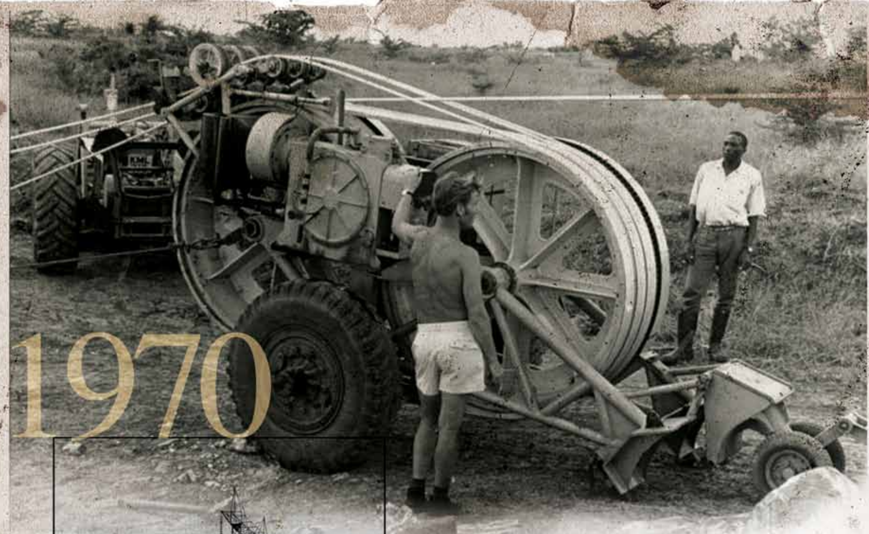
East Africa Power & Lighting Company technicians tensioning a line in 1970.
