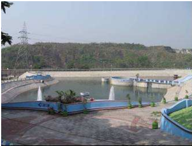
Photo: GREAT ROLE MODEL PROJECT - a Rain Water Harvesting (RWH) project implemented within the premises of manufacturing unit of Tata Motors at Jamshedpur
