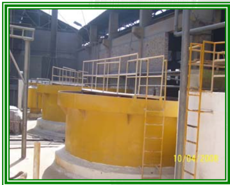
Clarifier of Effluent Treatment Plant
