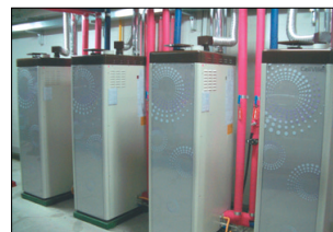
Onsite Installation of Fuel Cell Facility
