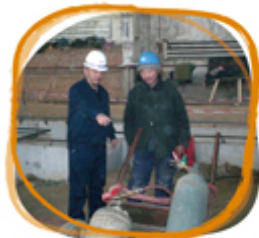
Staff of the Department of Work Safety Equipment correcting the violation of safety regulations of a contractor
