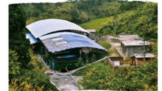
Xianglushan Sewage Treatment Station
