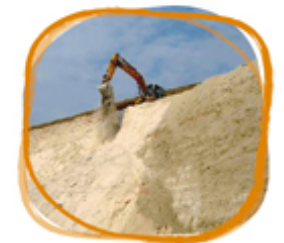
Excavator in slope-reducing operation on top of the slope
