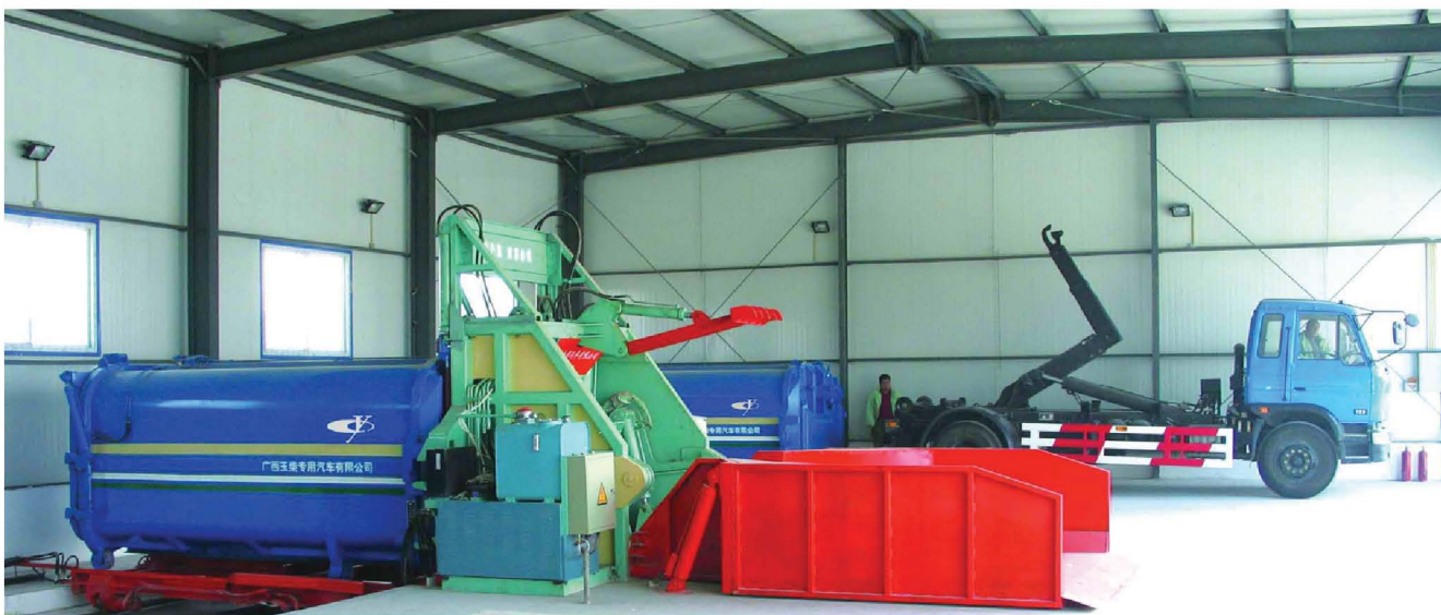
▲ Beijing-III garbage transfer station
