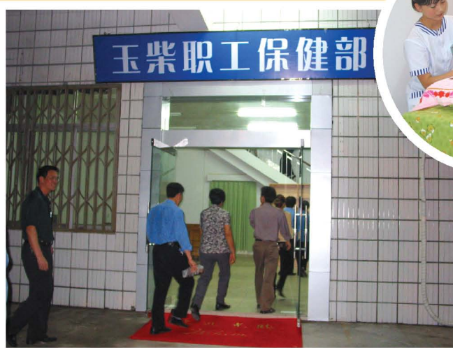
▲ Employee health care center
