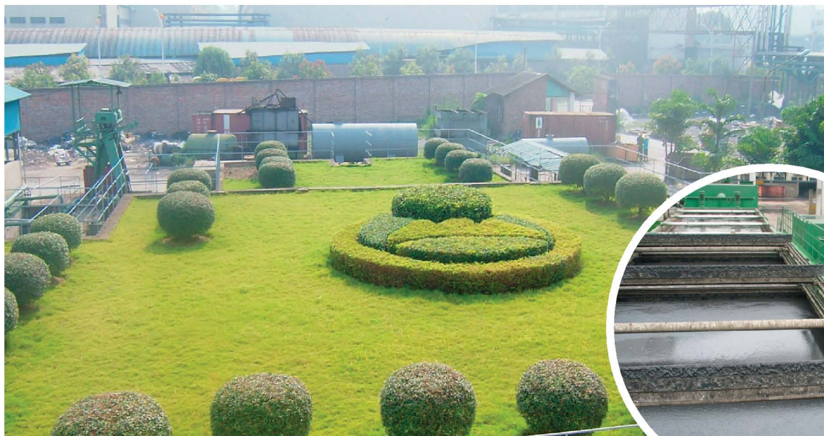
▲ cover of the regulating tank of the waste water disposal station
