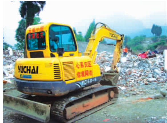
Rescue worker driving Yuchai Excavator to clear ruins
