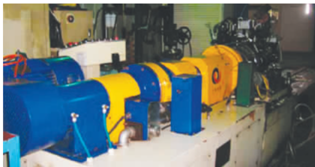
== Hot Running-in Bench Utilizing Nuclear Technology ==
