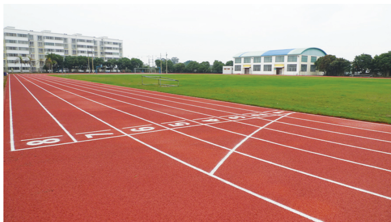
Brand-new plastic track in Yuchai Stadium
