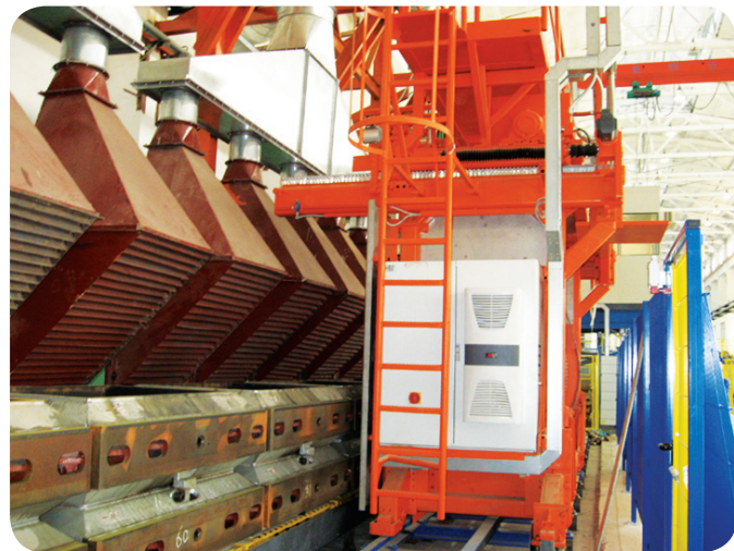
Automatic casting machine, the workers no longer have contact with high temperature ladle
