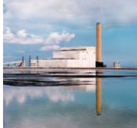
Lynemouth powerhouse, U.K.
