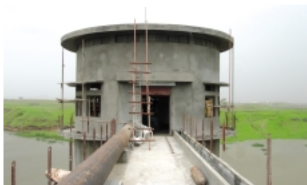
Nandurbar Water Supply Project
