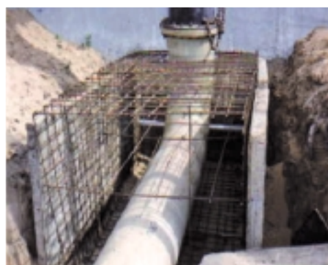
Laying of GRP Pipes, 2 x 125 MW, NLC
