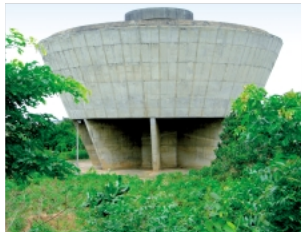
Lagos Water Supply Rehabilitation
