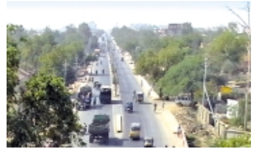
Newly Laid Road, Anjar
