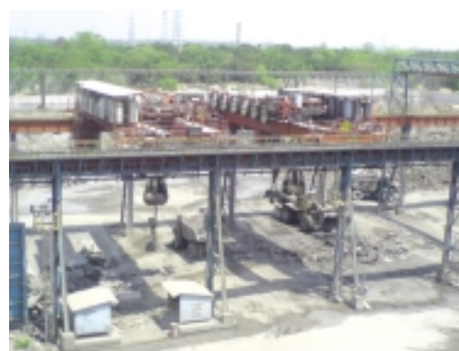
Waste Recycle Plant, Tata Steel Limited
