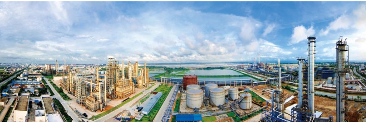
Sinopec Zhanjiang Dongxing Refining and Chemicals
