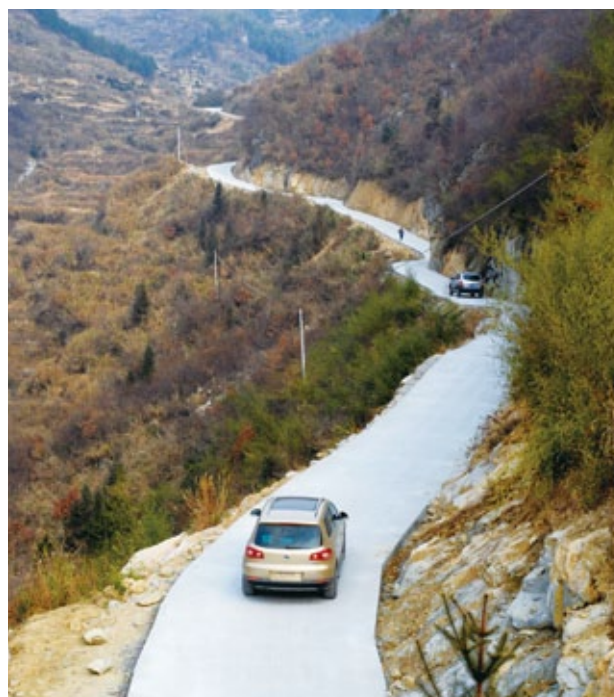
Road built by Sinopec in poverty-hit county
