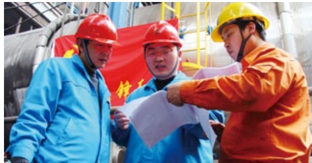
Sinopec employees discussing dryer maintenance issues
